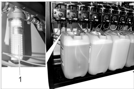
1 Filter for frost-protection pump
